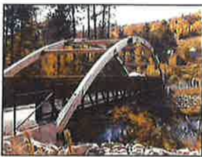
Mesabi Trail Bridge over Wynne Lake
